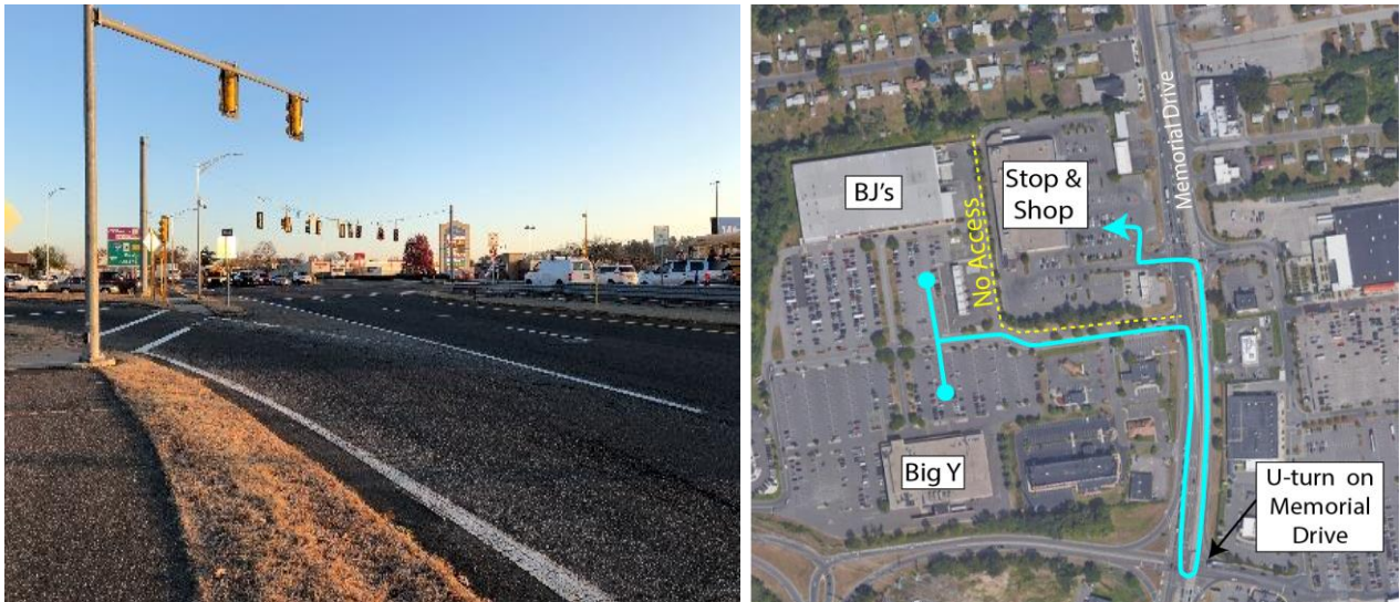
(Right) Lack of vehicular access between properties necessitates indirect travel patterns on Memorial Drive, which can lead to increased congestion and delay.
